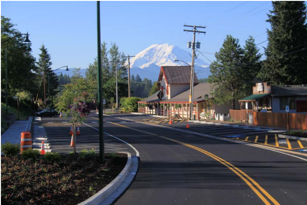
Railroad Ave Reconstruction Project 2010
