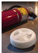
Smoke alarms should be replaced after 10 years of the date of manufacture. You can usually find the date on the back of the alarm once you remove it to change the battery. It is a good idea to replace the alarm every 10 years even if your alarm is hard wired into your home.
