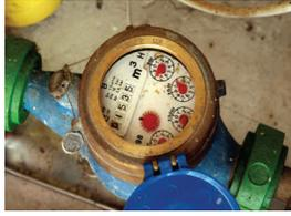
The new meters have the capability of being read electronically by radio signal. Once all of the meters have been replaced, this enhancement will save the City about a day-and-half of labor time each month as well as increased recording accuracy.
