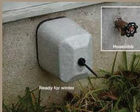
When it's cold, let hot and cold water trickle at night from a faucet on an outside wall; open cabinet doors to allow more heat to get to un-insulated pipes under a sink or appliance near an outer wall; make sure heat is left on and set no lower than 55 degrees; if you plan to be away: (1) Have someone check your house daily to make sure the heat
