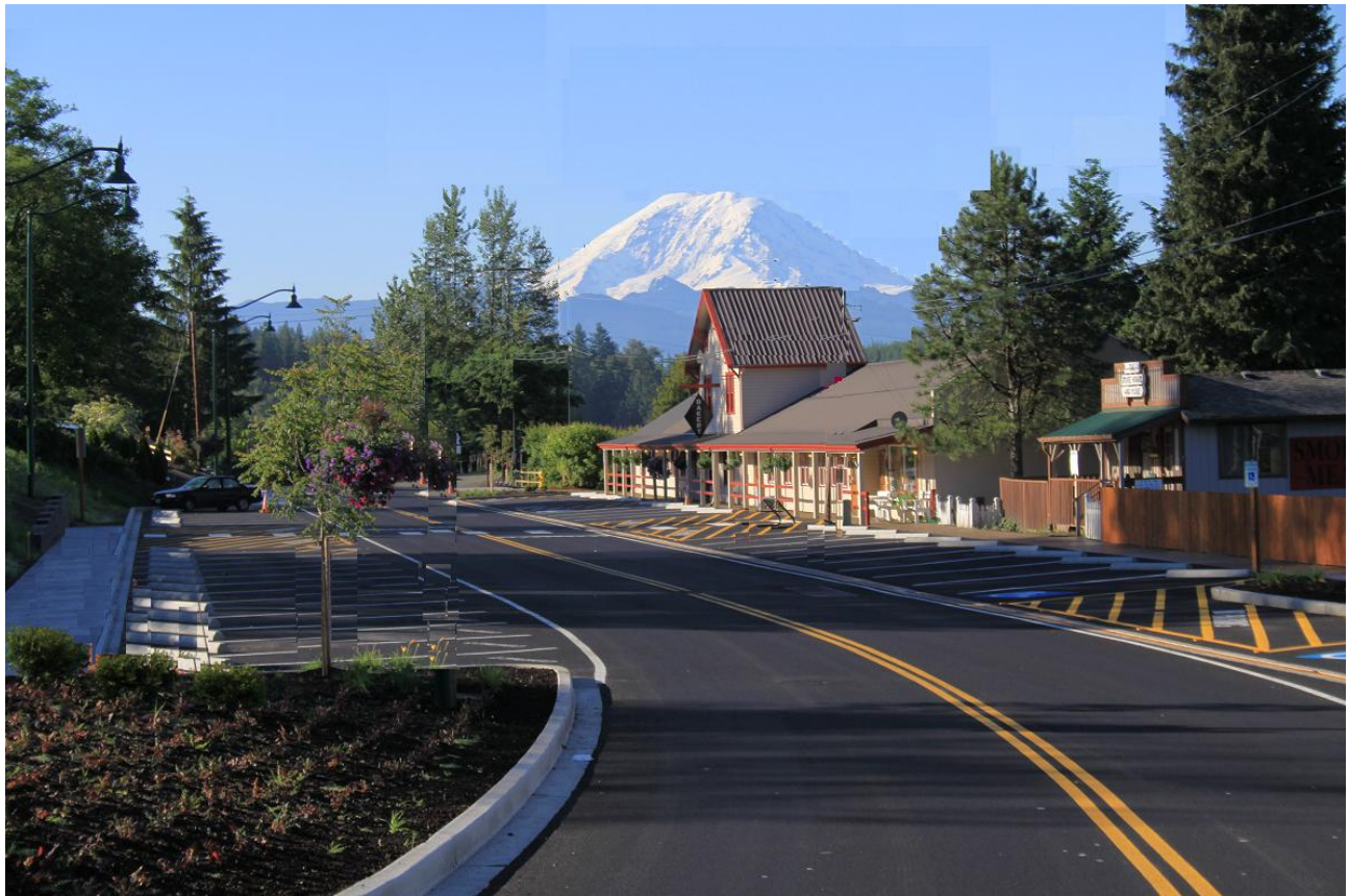
Railroad Avenue Project, completed in 2010
